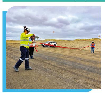
As part of our continuous improvement strategy, we built the **Teo Road,** a 1.2 km project located in the northern area of the west pit, designed with high engineering standards. The intervention included rigorous foundation ground improvement and the use of **triaxial geogrid**, which increased the infrastructure's load-bearing capacity.
